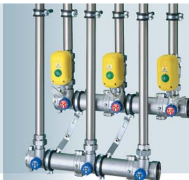
Start with zone valves
